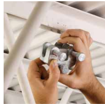
Step 2: Release thumb spring, allowing it to grip bar joist. Finger tighten the bolts to keep adaptor firmly in place.
