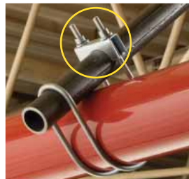
Step 5: Tighten bolts until heads shear off.
