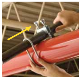
Step 2: Slide brace pipe over service pipe and through loops of the Quick Lateral Brace.
