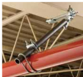
Step 4: Attach brace pipe to structure. (Pictured: I-Beam Adaptor with Universal Structural Attachment.)
